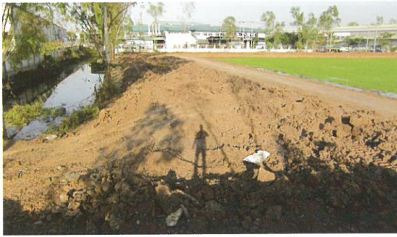
FIGURE 11. Removal of existing dike
