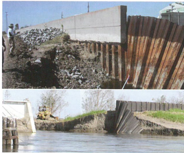
FIGURE 7. Examples of failed I-wall on levee after Hurricane Katrina (Photos Courtesy of ASCE)
