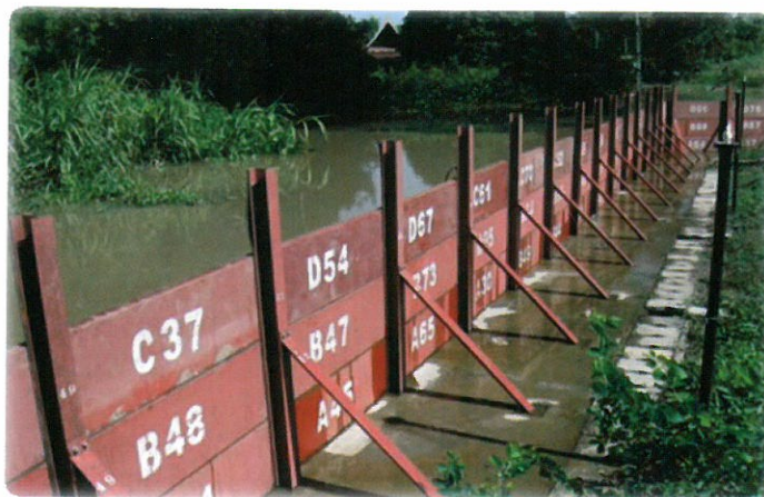
FIGURE 10. Example of Stop Logs Implementation at Bangsai, Ayutthaya
