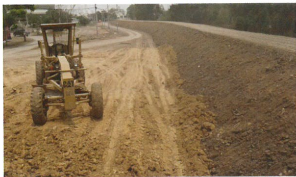
FIGURE 13. Soil compaction to required elevation (El. +4.40 m MSL.)
