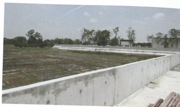
FIGURE 18. Completed RC Flood Wall
