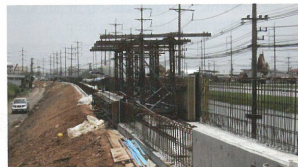
FIGURE 16. Preparation of Steel Reinforcement and concreting using slip formwork
