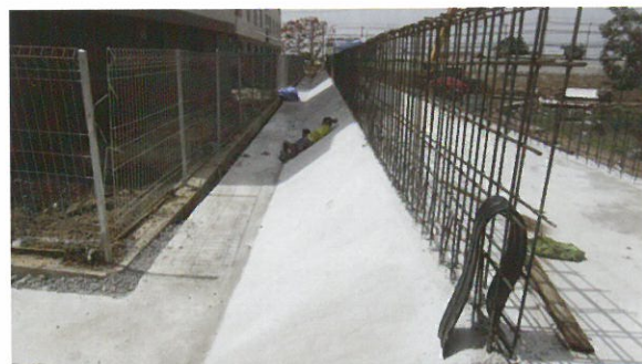
FIGURE 15. Concrete lining at side slope for erosion protection
