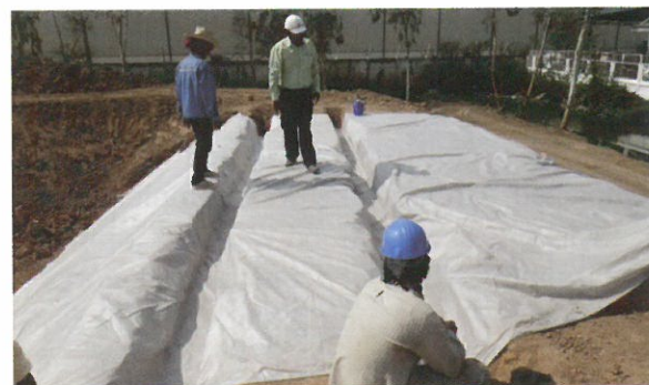
FIGURE 14. Trench excavation and spreading of geotextile before concreting
