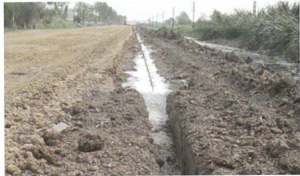
FIGURE 12. Construction of concrete cut-off trench to prevent seepage
