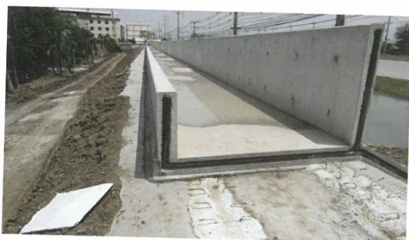
FIGURE 17. Water Stop at expansion joint of RC flood wall
