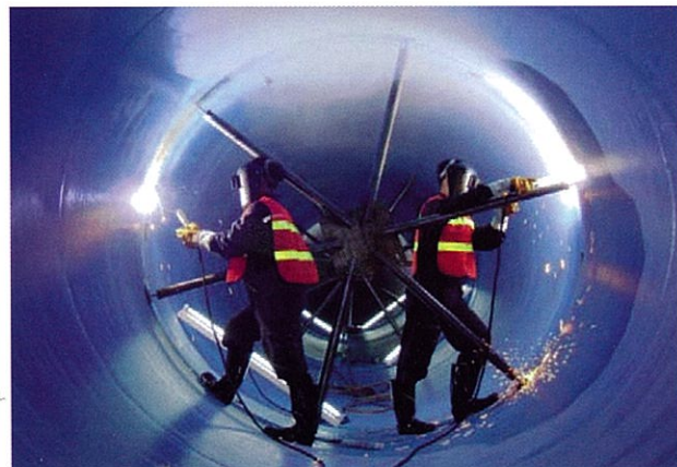
Tunnel inner lining installation MWA Water Transmission Tunnel
