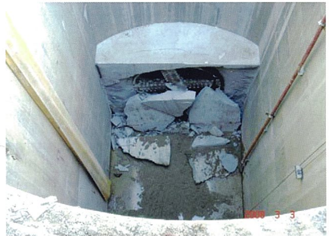
TBM Break-through to receiving shaft in the Water Transmission Project
