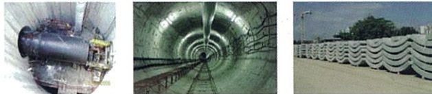
(a) Launching shaft (b) Flood drain tunnel (c) stock of precast tunnel segment
