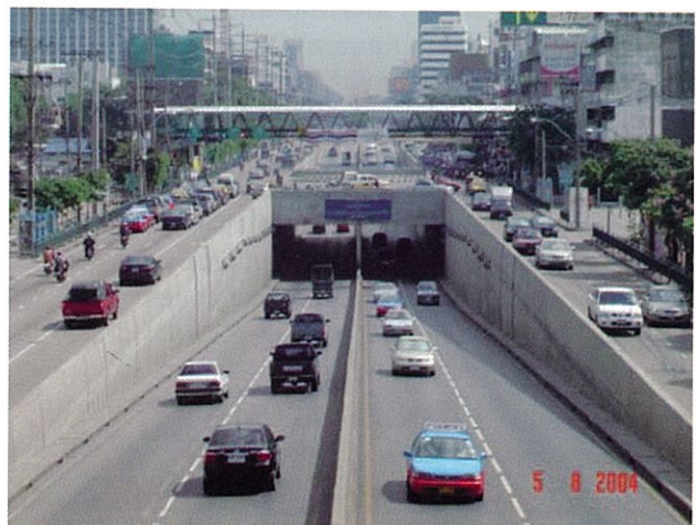
Underpass project constructed by diaphragm wall support cut-and-cover method (twin bored tunnels of the first Bangkok MRT is located underneath this underpass)
