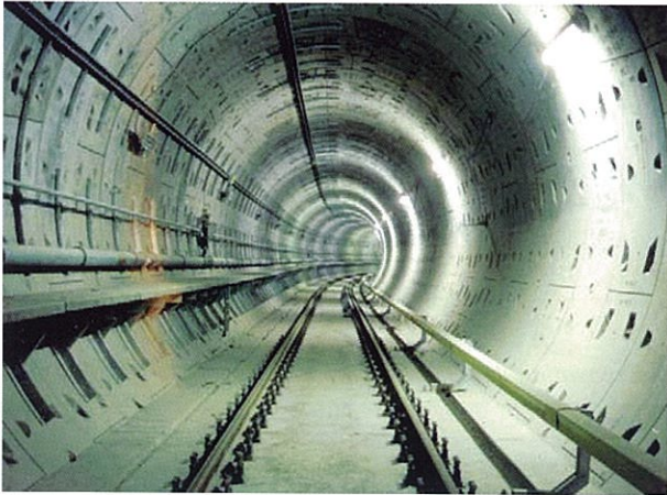
MRT first subway tunnel in Bangkok was constructed by EPB tunnel boring machines
