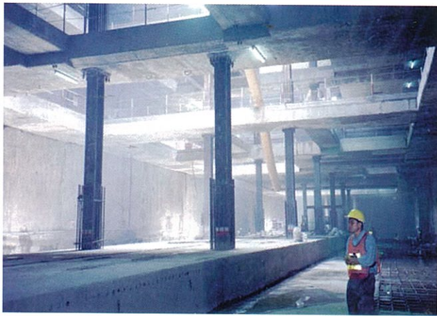
MRT Subway station box constructed by top-down method
