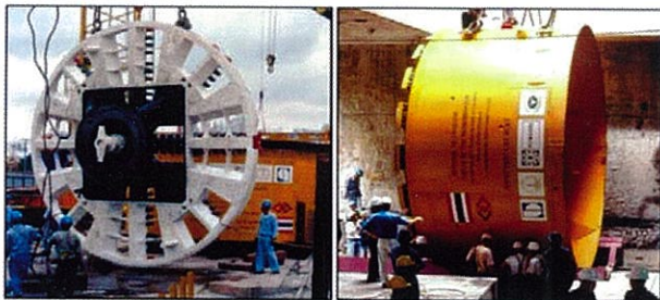
EPB Tunnel Boring Machine being assembled
